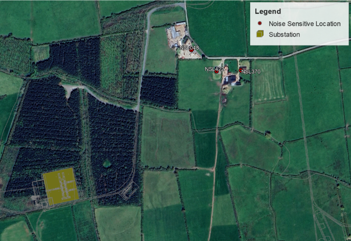
Figure 13-22: Location of substation compound
